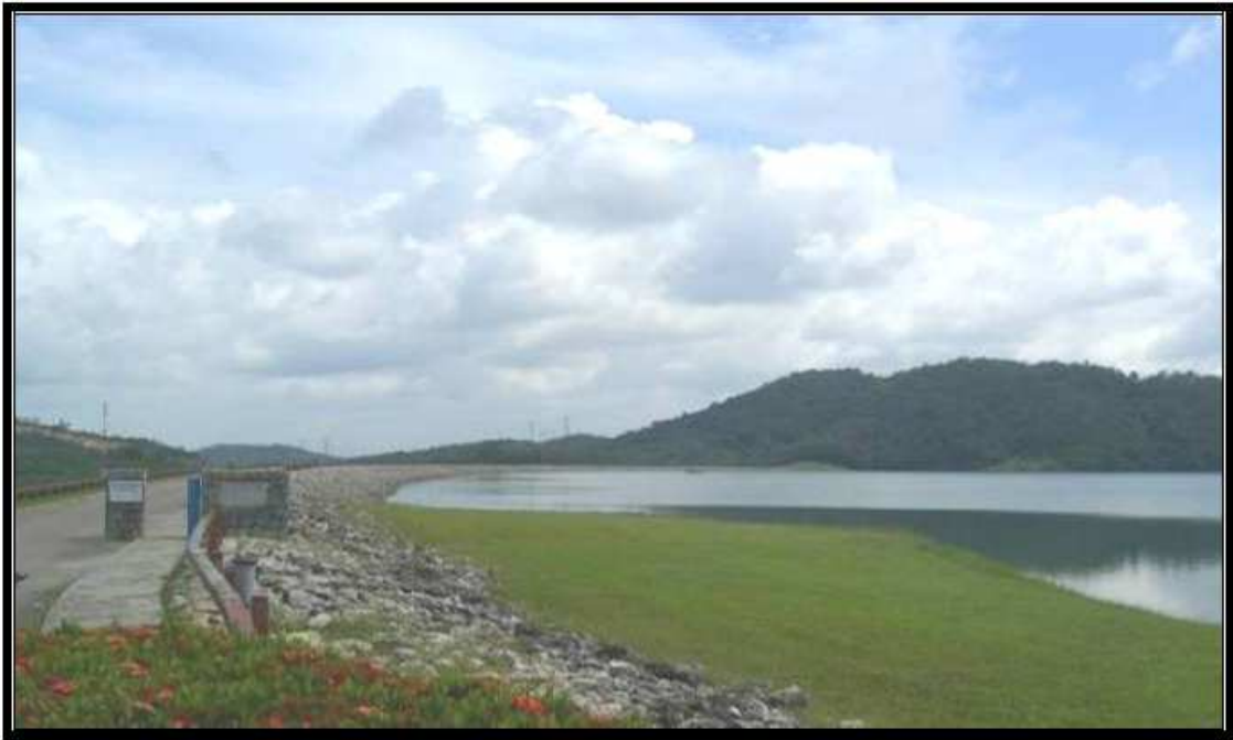
View of Existing Dam Crest
