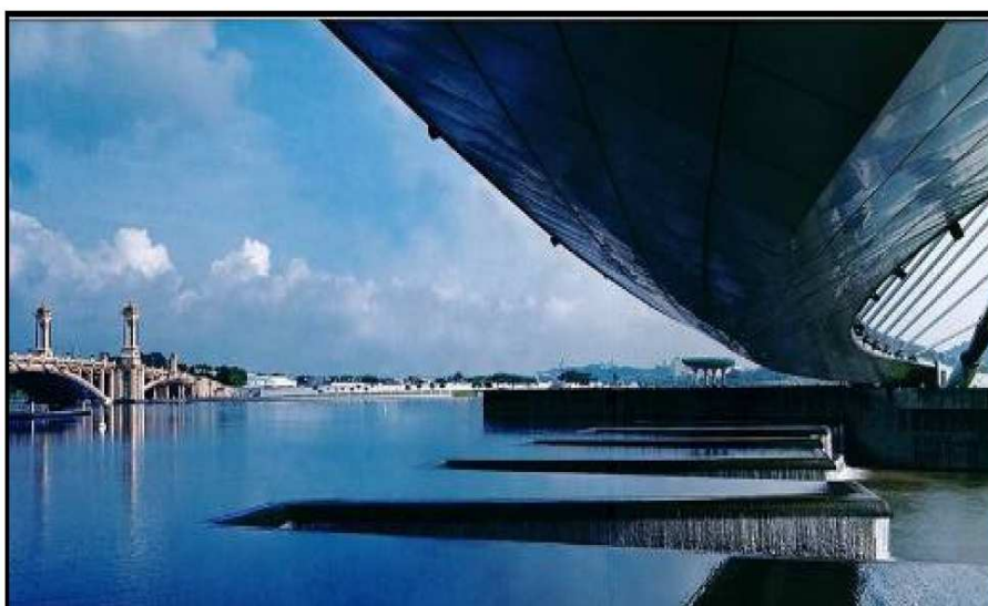
View of the Labyrinth Spillway at Putrajaya Dam
