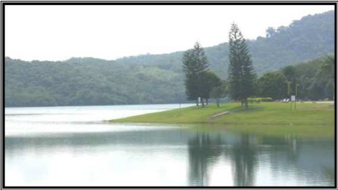
View of Existing Mengkuang Dam Storage Reservoir
