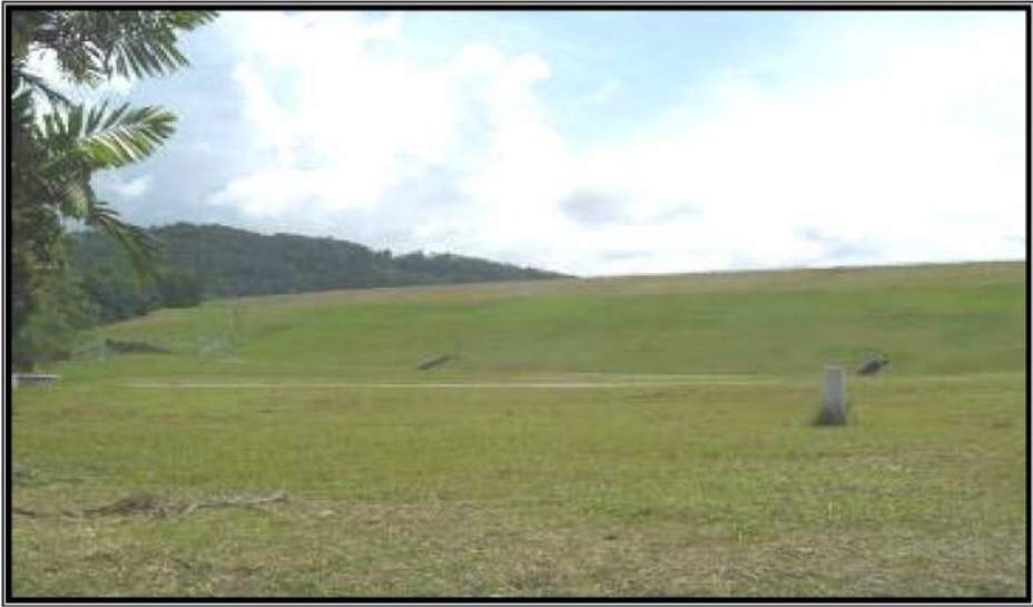
View of Existing Dam Embankment
