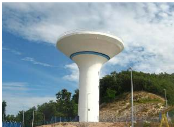
Rajah 7: 0.75JLH tangki elevated Bukit Bubus.
