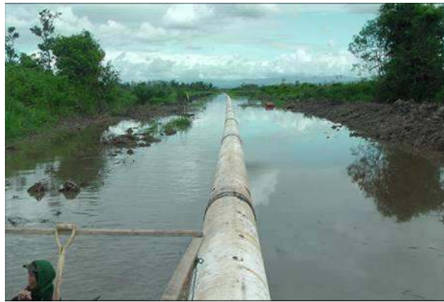
Rajah 14: Float - push & pull – sink method.
